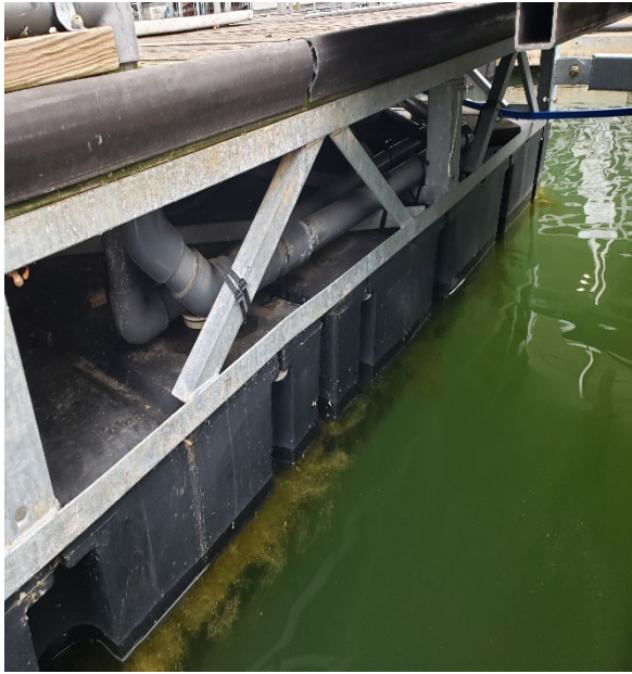
Photo Series #3. B&B's Cookson Bend Resort & Marina. April 10, 2021. Several hoses, tubing, pipes, and floating platforms had to be replaced due to deterioration over time.
