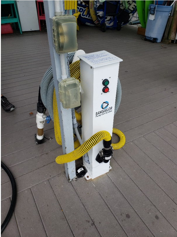
Photo Series #2. Serenity Point Resort Marina, LLC July 12, 2021 Pump-out Station with vacuum hoses and piping to the main unit
